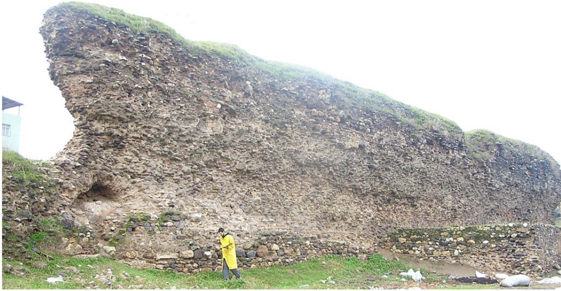
Fig. 3. The City Walls, north section
