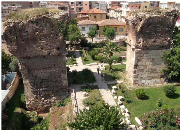
Fig. 11. The Church of St. Ioannes, NE and NW piers from North
