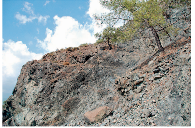
Res. 5 Phaselis-Olympos yolu ve istinat duvarı Fig. 5 Phaselis-Olympos road, and the defensive wall
